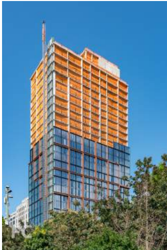
Southwest corner of 50 Bridge Park Drive.
