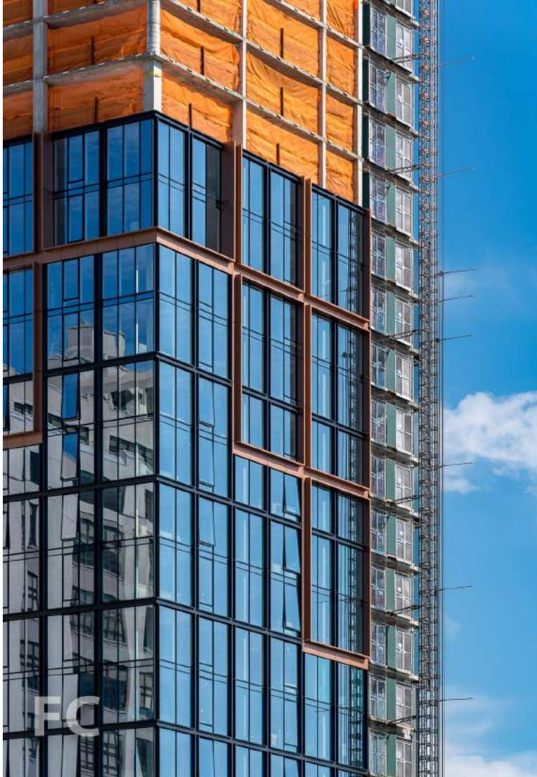
Close-up of the northwest corner of 50 Bridge Park Drive.
