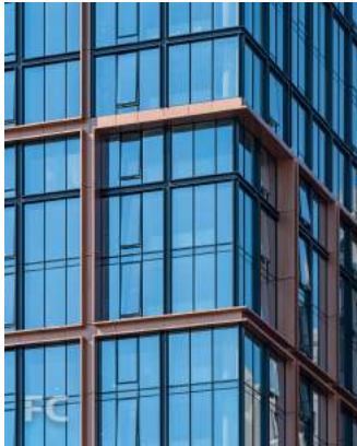
Close-up of the southeast corner of 50 Bridge Park Drive.
