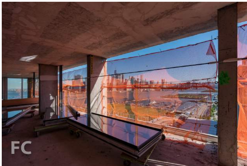
Curtain wall panels awaiting installation at 50 Bridge Park Drive.
