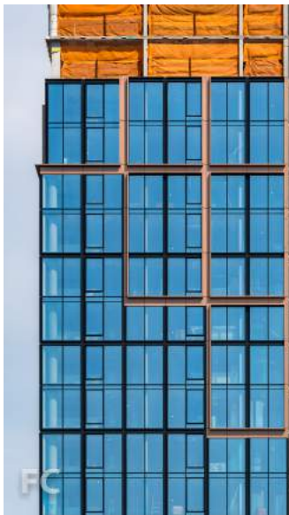
Close-up of the west facade of 50 Bridge Park Drive.
