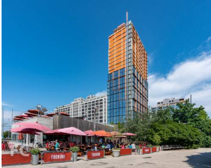
Southwest corner of 50 Bridge Park Drive.
